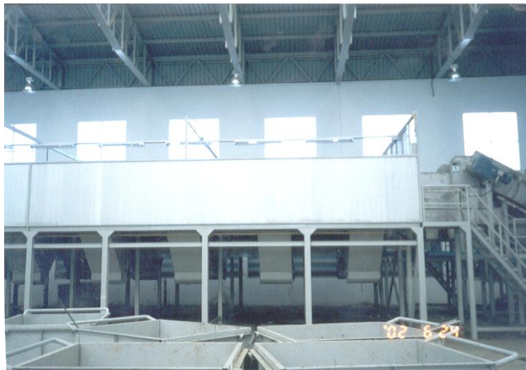
1 st MAZZANINE 16 HOPPER BOXES / 32 PERSONS WITH TWO “DOS” SORTING CONVEYOR
