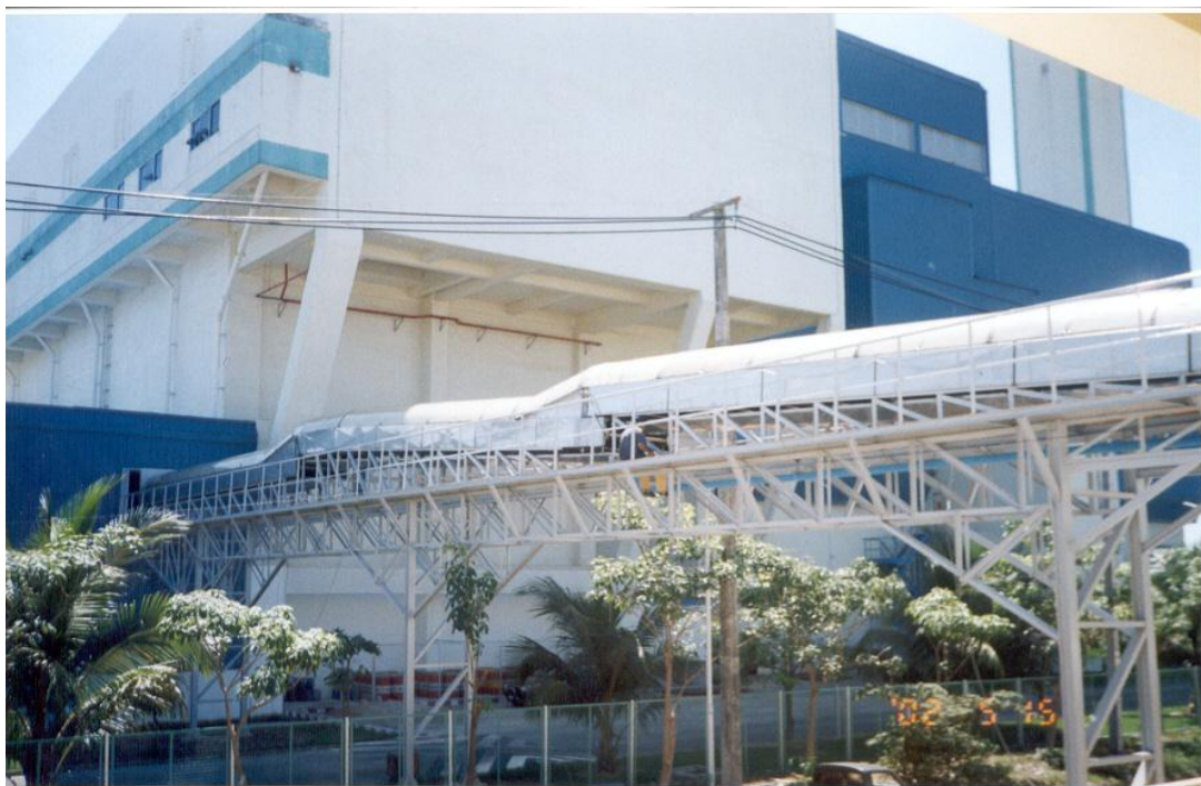
WASTE OUTFEED WITH “DOS” TUNNEL CONVEYOR TO INCINERATOR PLANT
