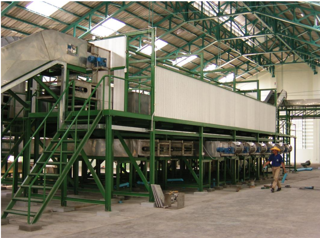
SORTING MEZZANINE AND RECYCLE CONVEYER
